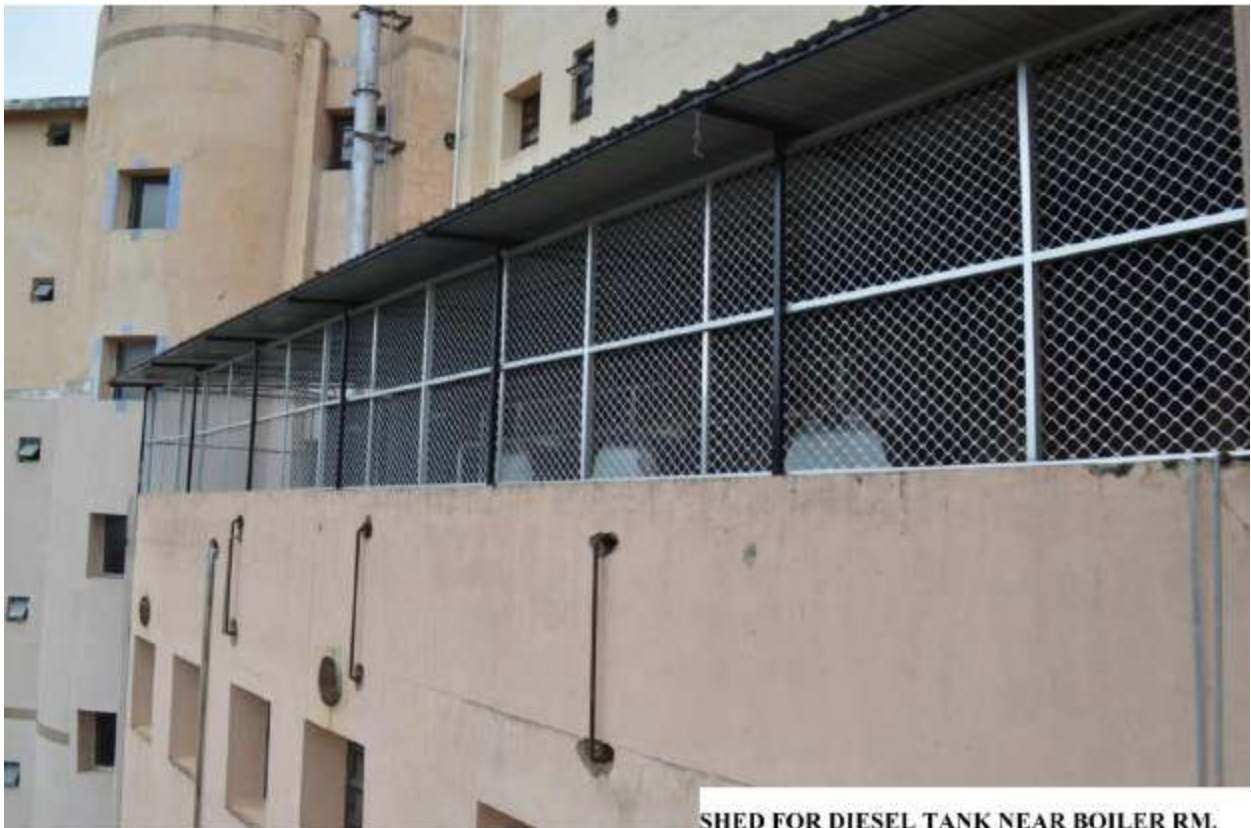
SHED FOR DIESEL TANK NEAR BOILER RM.
